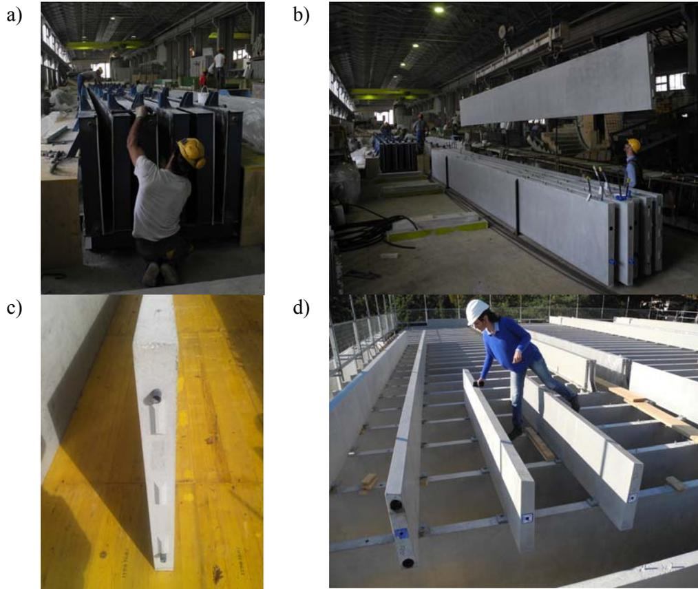
Figure 4: a) arrangement of steel formwork, b) handling of the 10.50 m elements, c) match-casted joint for the 21 meter beams and d) erection of longitudinal stiffeners over the transversal beams
